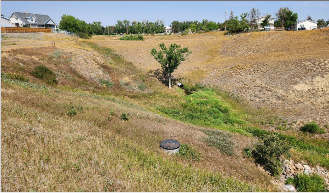
Photo 5: Culvert Upstream of the Tributary Coulee.
